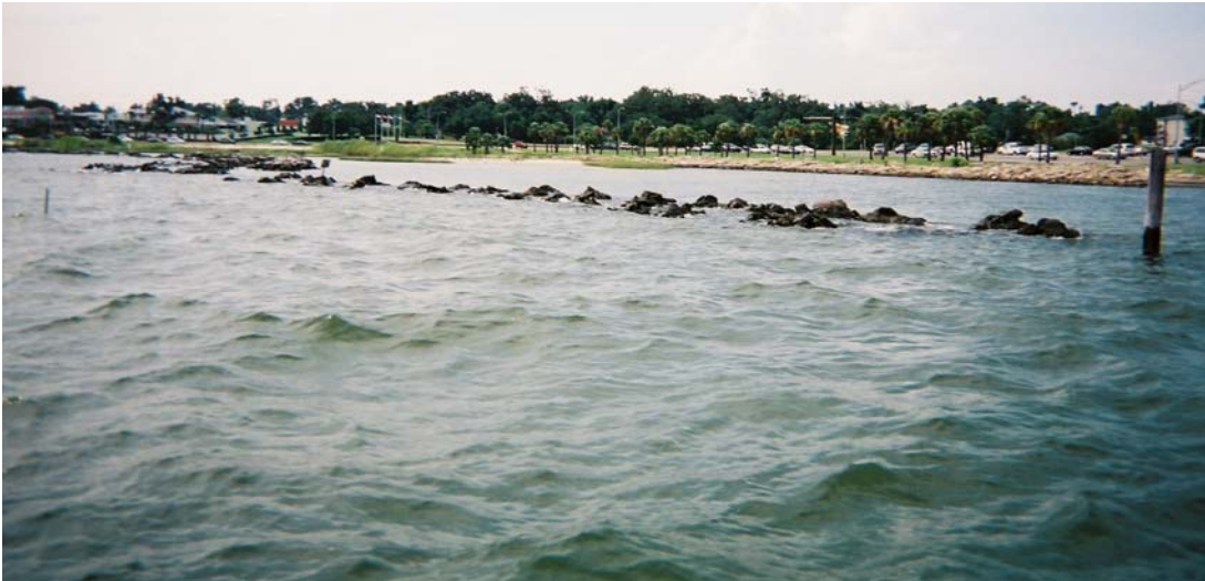
Figure 4. Visual comparison of the wave conditions seaward and landward of the structure.
