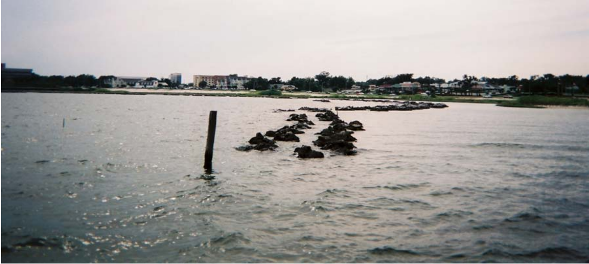
Figure 5. Wave propagation through the gap between the structure and the seawall (beyond the bottom of the picture). Note the reflected waves propagating nearly parallel to the structure.
